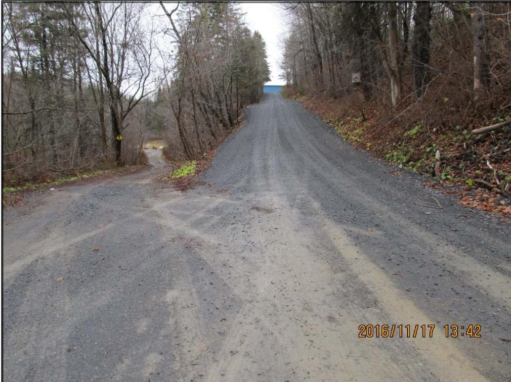
Public works access road after removing berms and adding geotextile and gravel to super-elevate the road. Reshaped ATV trail and used large rocks to restrict ATV access.
