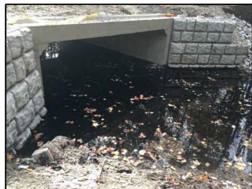
Kala Lane - The Town replaced two undersized culverts with a concrete box culvert with natural bottom.
