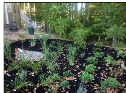
This rain garden infiltrates and filters roof runoff, and has allowed an adjacent eroding area to stabilize.
