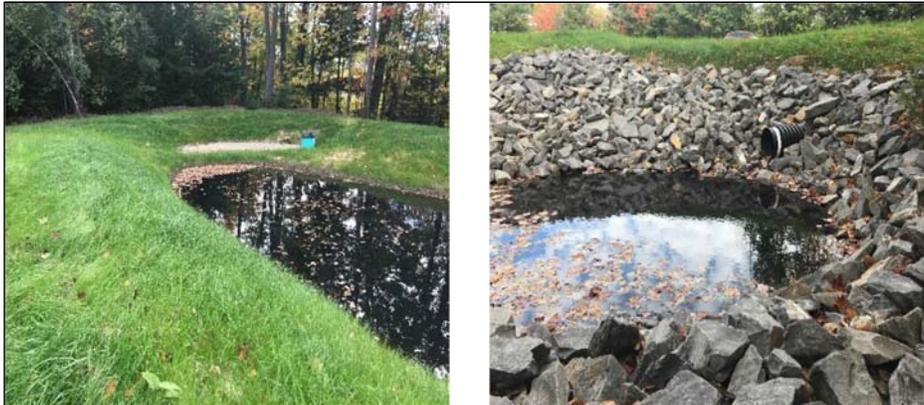
The La-Z-Boy stormwater pond next to Red Brook was rebuilt with a gravel bench and outlet step pools (right) to reduce stormwater and downstream habitat impacts.
